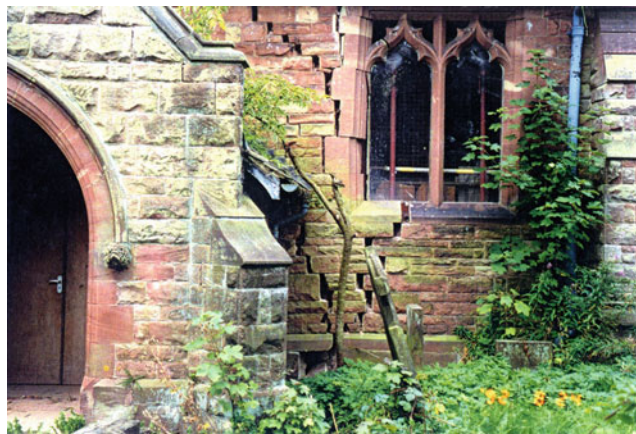
Mining Subsidence Induced Fault Reactivation, Figure 5 Barlaston church, Staffordshire, UK, was severely damaged by mining-induced fault reactivation. (Photograph © Laurance Donnelly).
