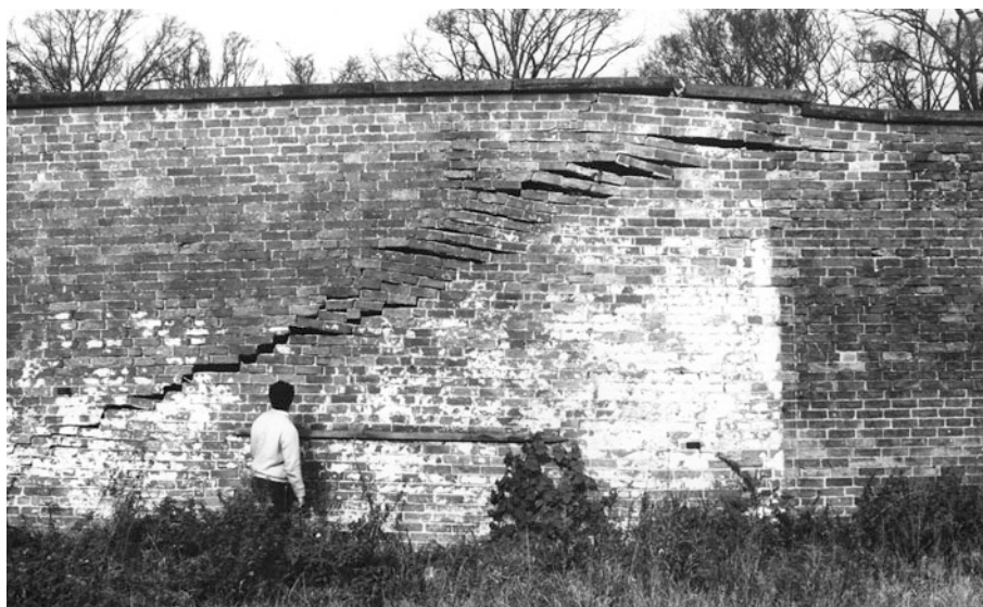
Mining Subsidence Induced Fault Reactivation, Figure 4 Compression to a 5.0 m high retaining wall, caused by fault reactivation and subsidence, Eastwood Hall, Nottinghamshire, UK (Photograph after Whittaker and Reddish, 1989).
