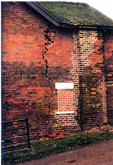
Mining Subsidence Induced Fault Reactivation, Figure 3 Damage to houses caused by the mining-induced reactivation of the Hopton Fault, Oulton, Staffordshire, UK (Photograph © Laurance Donnelly).
