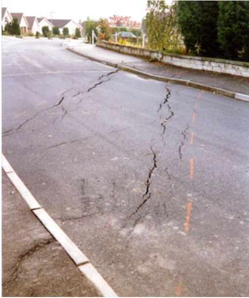
Mining Subsidence Induced Fault Reactivation, Figure 6 Reactivation of the Inkersall Fault, Derbyshire, generating a graben, which caused widespread damage to two schools, houses, roads, and walls in the late 1980s and 1990s (Photograph © Laurance Donnelly).
