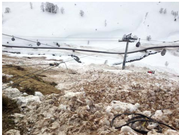
Figure 9. View of the tower taken from above on 18 February 2013. A wire was stretched to stabilize the tower pushed over by the sliding slab. Courtesy of J.-L. Pons.
