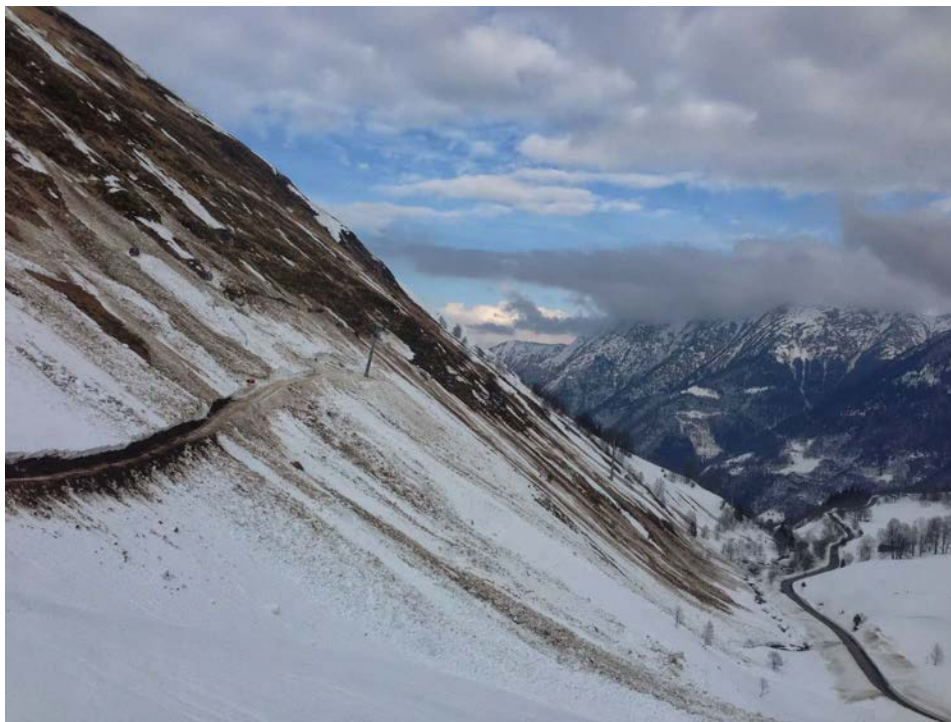
Figure 7. Side view of tower P10 on 18 February 2013. The glide crack is about 60 m above the tower. A track was dug for the rescue operation. Courtesy of J.-L. Pons.
