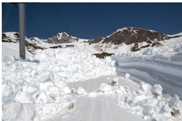
Figure 3. Tower hit by the avalanche (with no damage) and left-hand border of the avalanche track for the Lauzière chairlift at Saint-François-Longchamp.
