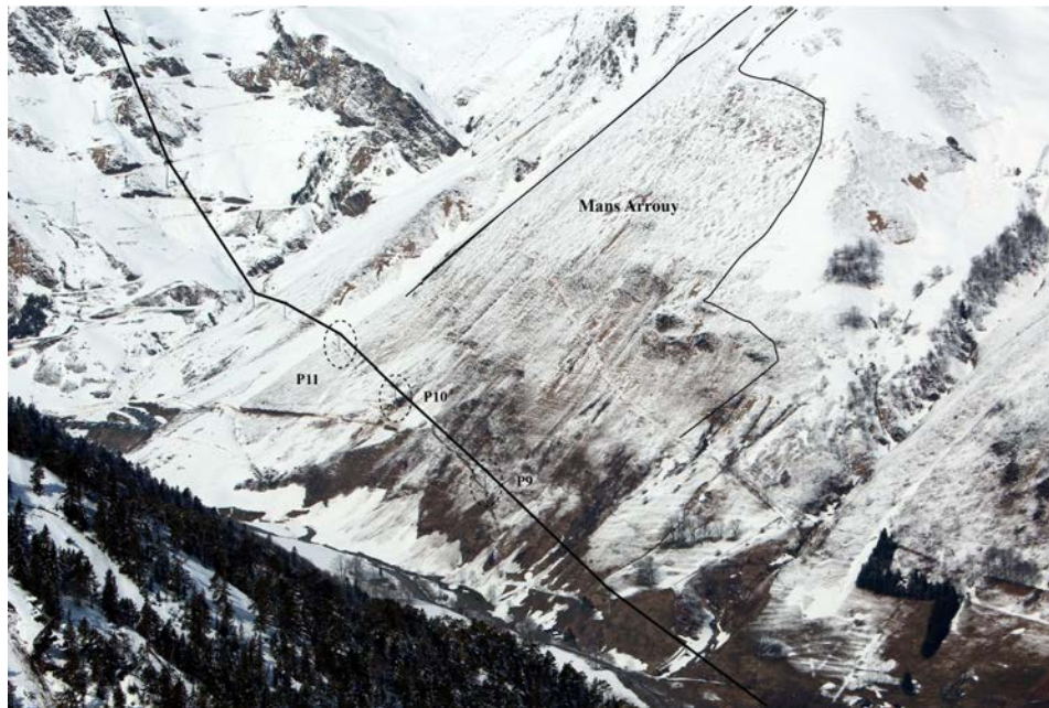
Figure 6. View of the site in late spring 2013. Snow deposits at the toe of the Mans Arrouy slopes are still visible. Tower P10 was the one damaged by gliding snow on 16 February 2013.
