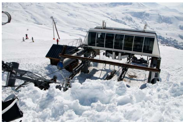
Figure 4. Lower station hit by the glide avalanche at Saint-François-Longchamp.
