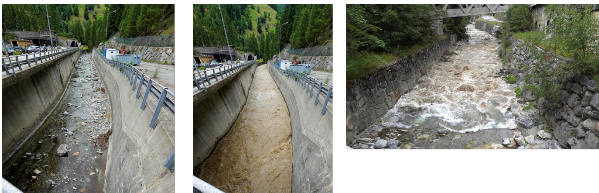
Figure 1. On the left before the gate opening, in the middle during the opening of the bottom gate. On the right, the wave passing through, with the sediment load change clearly visible.
